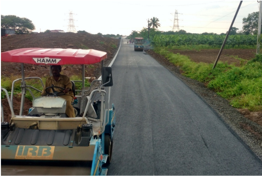
Service Road completed in Sindaphal
