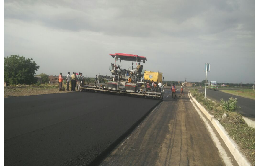
Four laning completed in Ule village
